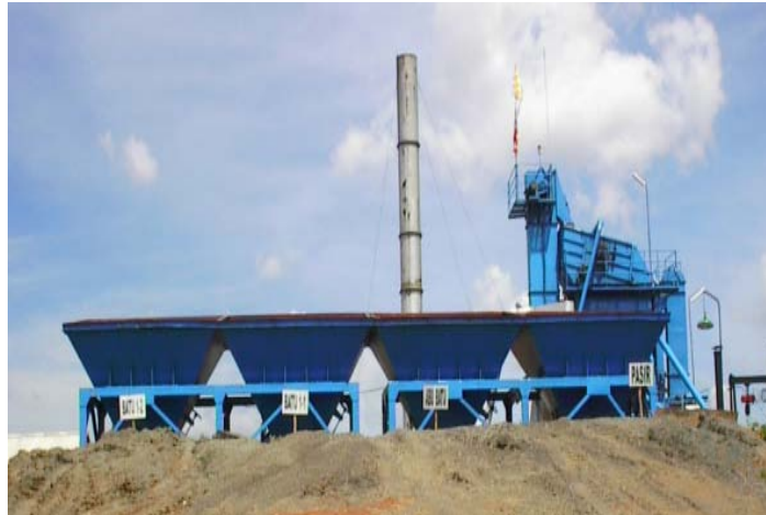
Gambar 2.10. Asphalt Mixing Plant
